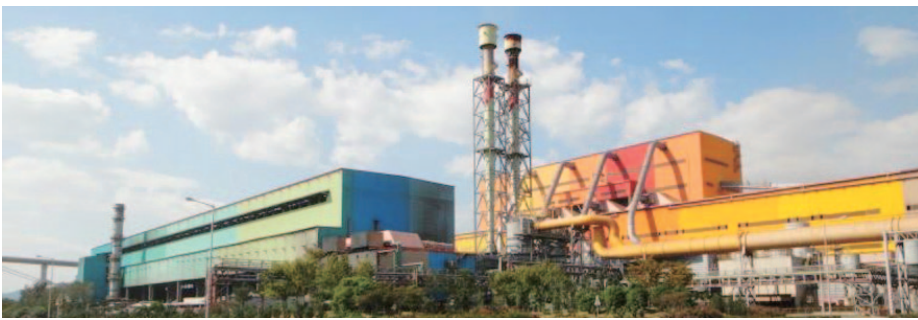
Figure. 1 Site overview of Gwangyang No.4 Hot Strip Mill Plant Project, POSCO (steel making plant)
